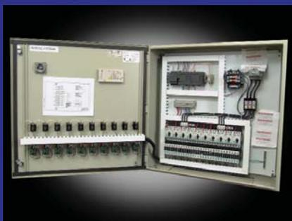
A typical motor control panel with the temperature controller for the Tower Tech 10-fan Modular Cooling Tower
